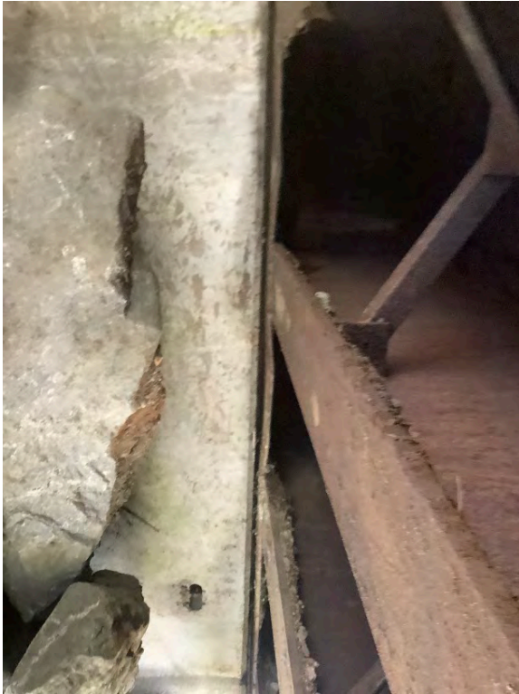
Right Bank Abutment when facing downstream
