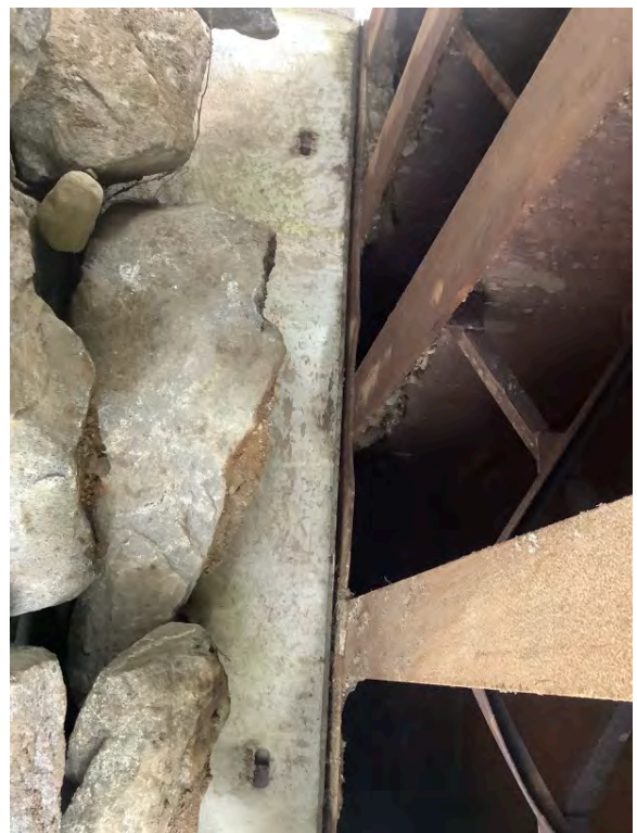
Right Bank Abutment when facing downstream
